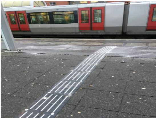
Plug/ schroef-en-ring verbinding in betontegels.
